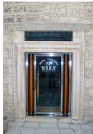
22 Projekt 24: portal nakon radova Project 24: portal after restoration
