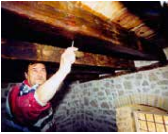
13 Projekt 13: u tijeku radova Project 13: during restoration
