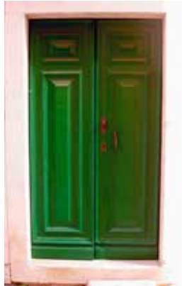
30 Projekt 40: jedne vratnice nakon radova Project 40: doors after restoration
