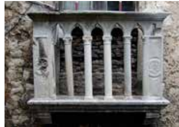
20 Projekt 21: stanje balkona nakon radova Project 21: condition of balcony after restoration
