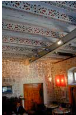
14 Projekt 13: stanje stropa nakon radova Project 13: condition of ceiling after restoration
