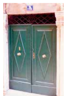
12 Projekt 11: vratnice iz 19. stoljeća nakon radova Project 11: 19th-century doors after restoration
