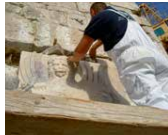
28 Projekt 37: montaža grbova Project 37: installing of coats of arms
